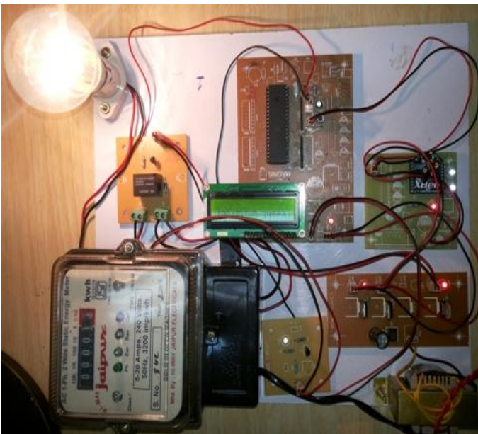
Fig.8. Hardware module of Energy Meter 1 at User end.
