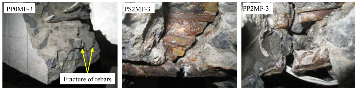
Fig. 7. Details of failed cross-sections in fatigue tests.
