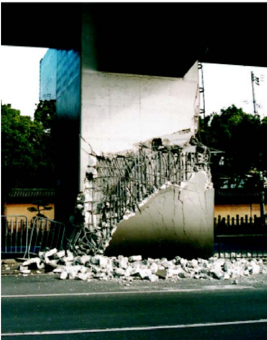
Fig. 1. Shear rupture of the piles Hanshin-Awaji seism [8].
