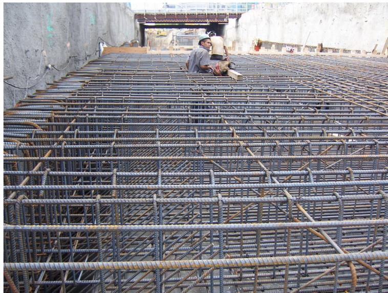
Figure 8 Roof Slab and Wall Reinforcing
