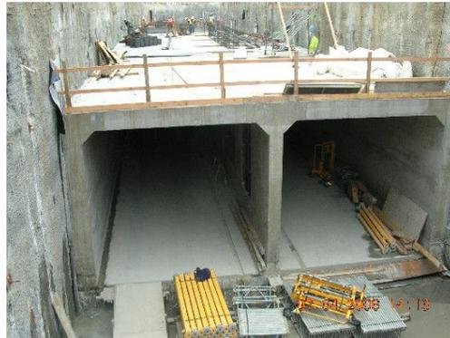
Figure 7 Roof Slab of Side-by-Side Box
