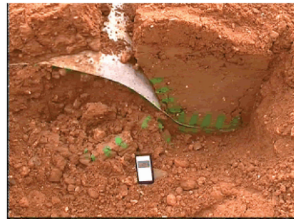
Figure 11. Failure of trapezoidal trench in flint clay.
