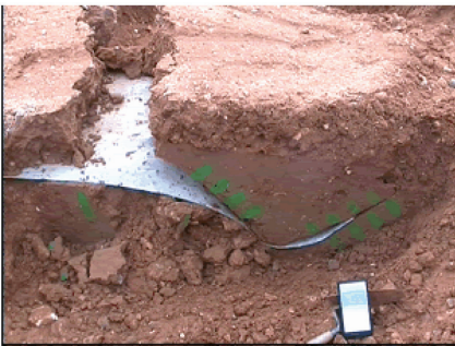
Figure 10. Failure of V-shaped trench in flint clay.
