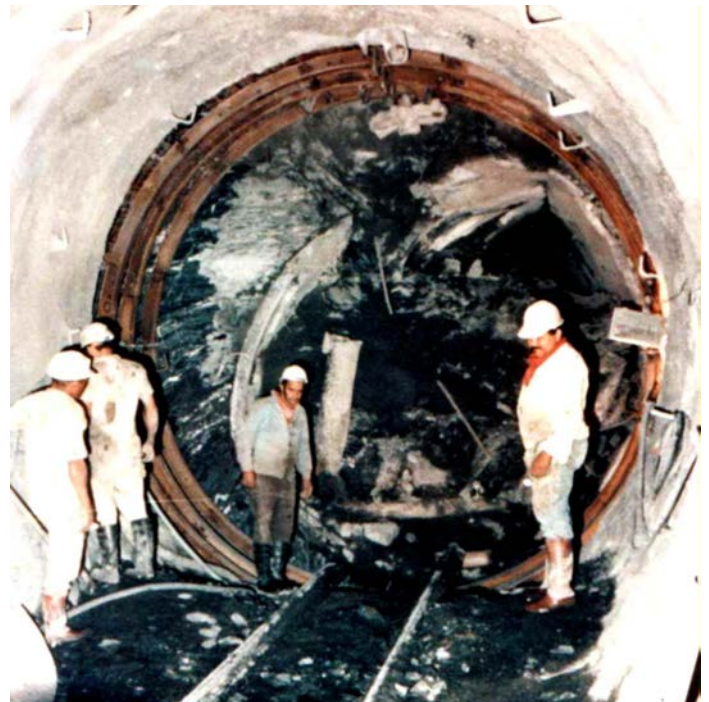
Fig. 8: Yacambú-Quibor tunnel in Venezuela. Mining out the remains of a tunnel boring machine trapped by squeezing of the tunnel during a stoppage of the drive.
