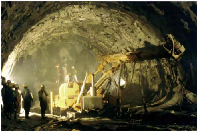
Fig. 10: Drilling unit for the installation of 12 m long 75 mm diameter pipe forepoles to form a protective umbrella under which the headrace tunnel was successfully mined through the fault zone in the Nathpa Jhakri headrace tunnel.
