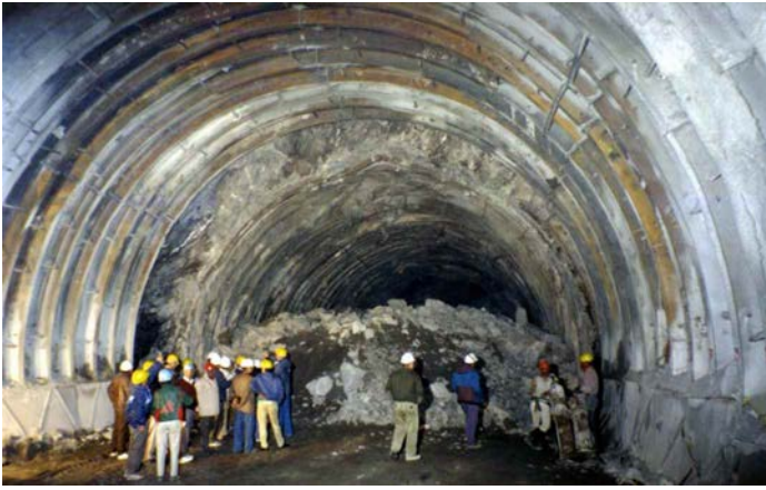
Fig. 9: Severe squeezing in a fault zone encountered by the 10 m span top heading of the headrace tunnel for the Nathpa Jhakri hydroelectric project in India.
