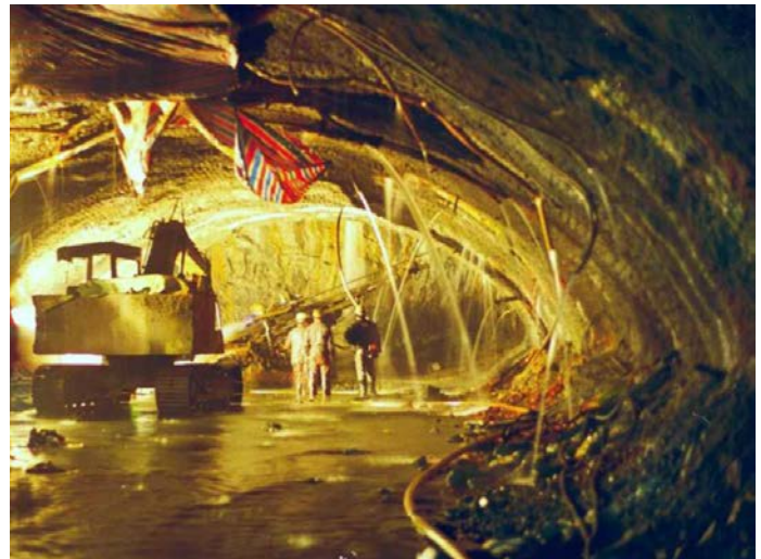
Fig. 22: The occurrence of large volumes of water can give rise to difficult construction problems in tunnels.
