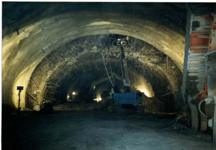
Fig. 11: Re-mining the perimeter of the 16 m span Mucha tunnel in Taiwan after severe squeezing in a fault zone. Photograph reproduced with permission from Sinotech Engineering Consultants Inc., Taipei.
