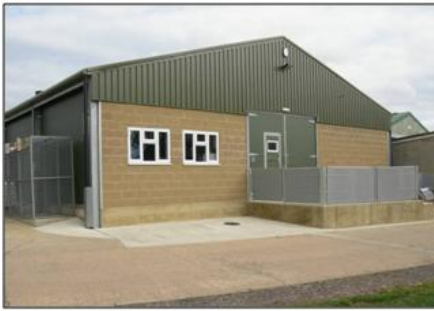
The new, BBSRC-funded, welfare barn at the Royal Veterinary College. It comprises two full-sized sections of a typical livestock building and ten environmentally-controlled rooms, each holding about 250 broiler chickens or 20 finishing pigs. It was built in 2005 at a cost of £600k and is currently being used for research on PLF.
